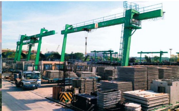
Precast Yard in Singapore
